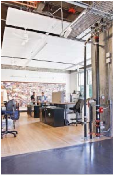
Shattuck Hall reopened in fall 2008 after a $9.35 million renovation. Built in 1915, the building's mechanical, electrical and structural systems are now exposed. (Photo courtesy PAE Consulting Engineers)
